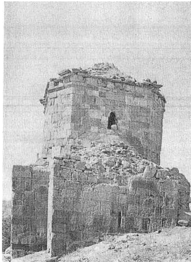
FIG. 4. A pre-twelfth-century Syrian church at Korluca, one of the monuments surveyed in the Keban Dam Salvage Project.
