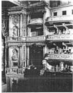
FIG. 5. A detail of the proscenium and boxes in the auditorium (c. 1900).
