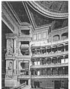
FIG. 6. Part of the auditorium during the reconstruction (1982).
