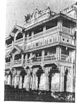
FIG. 12. Street elevation of the Ithnashiri Dispensary.
