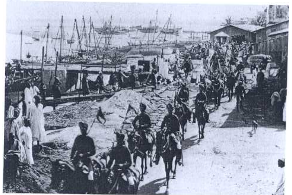
FIG. 5. The foreshore anchorage depending on the height of the tide before the construction of the new wharf.
