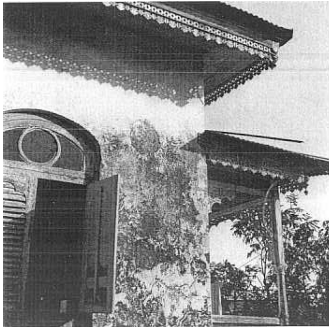
FIG. 17. Fret work fascias, iron railing and other details of mainly European influence.
