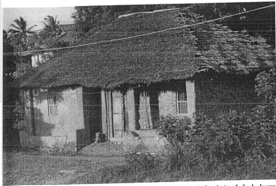
Fig. 7. Traditional 'Swahili house' in 'wattle and daub' construction with thatched makuti roof of palm leaves.
