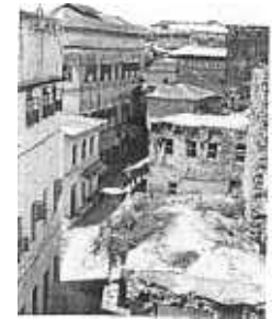
FIG. 20. Characteristic townscape with collapsed buildings.
