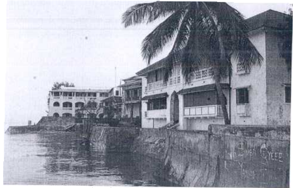
FIG. 19. Buildings of early twentieth-century origin facing the seashore.
