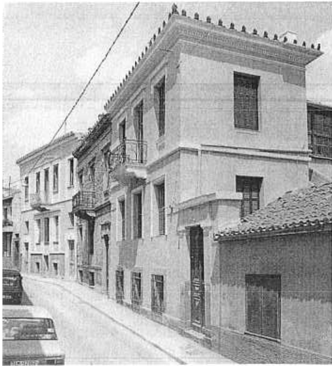
FIG. 9. A view of Tripod Street with restored houses flanking a decayed example.
