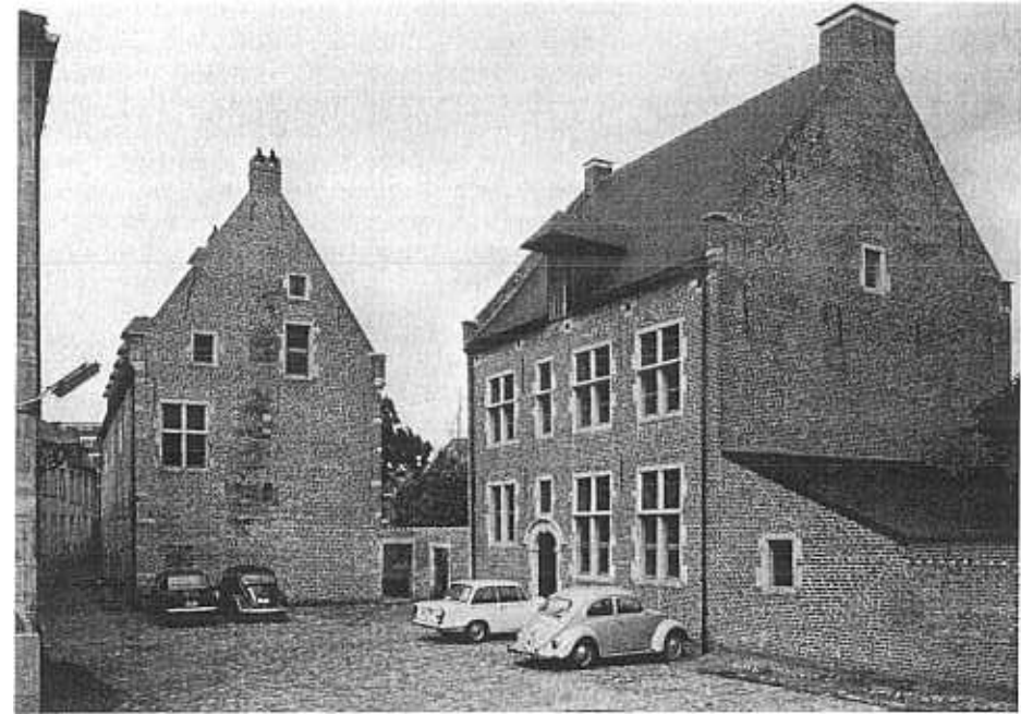
FIG. 11. The Grand Béguinage, Louvain; one of the houses restored as a staff residence. Note the exposed brickwork and renewed windows.
