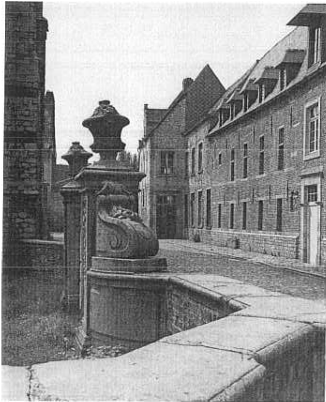
FIG. 12. The Grand Béguinage, Louvain; the new windows are clearly distinguishable by the omission of mullions and transoms.
