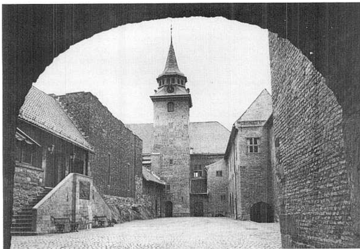
FIG. 10. The courtyard seen from the north with the new East Wing finished in 1963.
