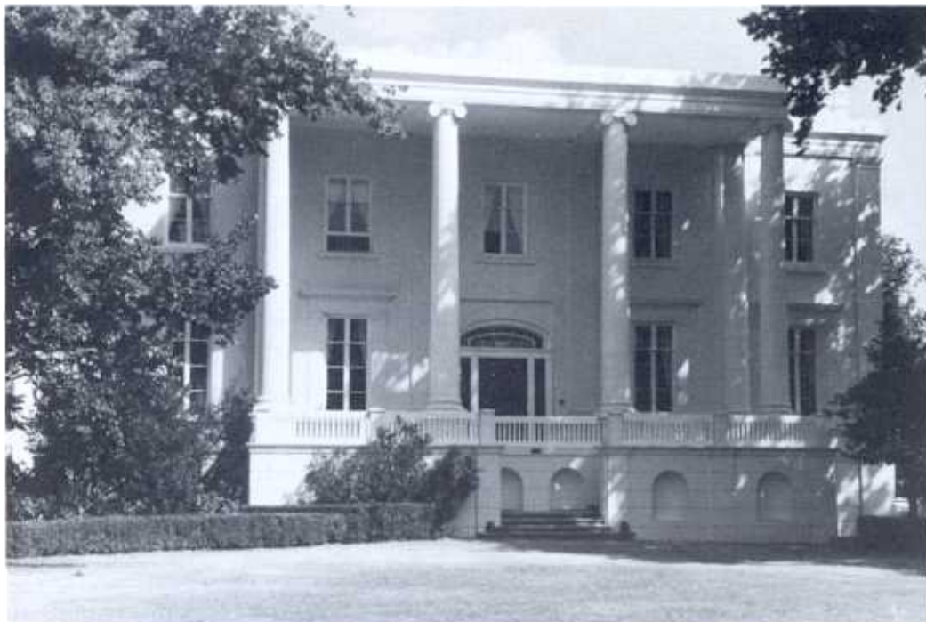
FIG. 12. Clarendon, Tasmania after the reconstruction of the portico in reinforced concrete ( Clive Lucas ).
