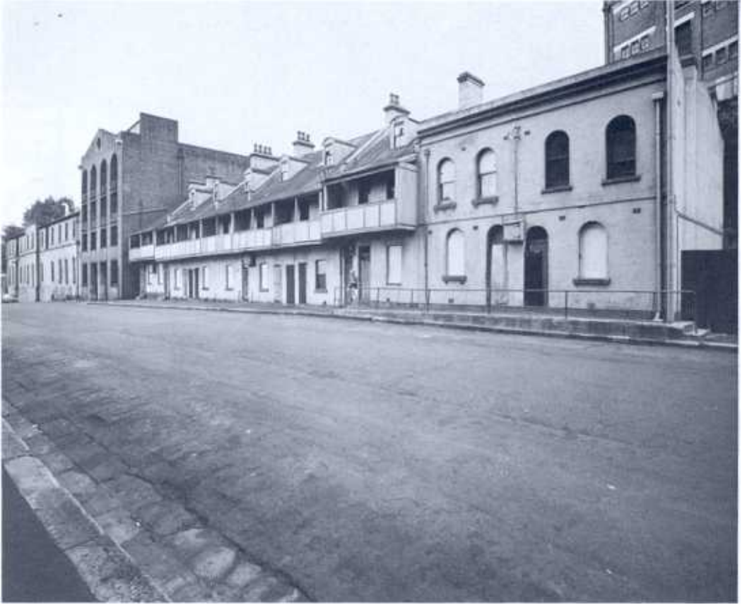
FIG. 10 .3–31 Playfair Street, The Rocks, Sydney, NSW before restoration ( Tim Collis-Bird )
