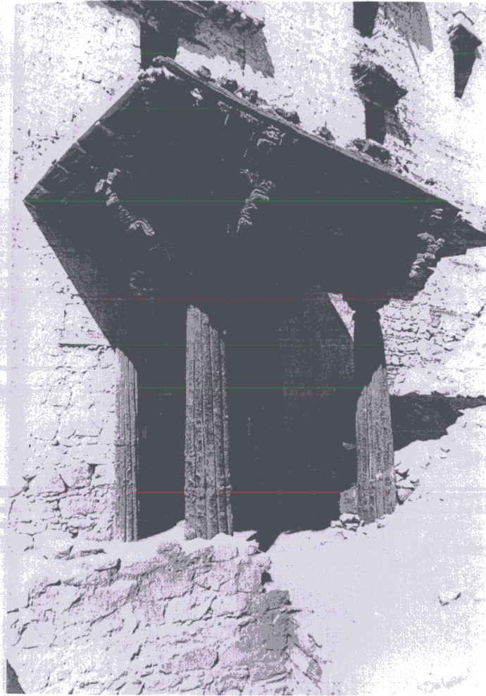
FIG. 12. On the eastern side of the palace the main entrance porch has an unusual canopy constructed of elaborately carved timber. Probably of Kashmiri influence, it depicts the Snow Lion which was the king's emblem. (Photo by John Sanday.)
