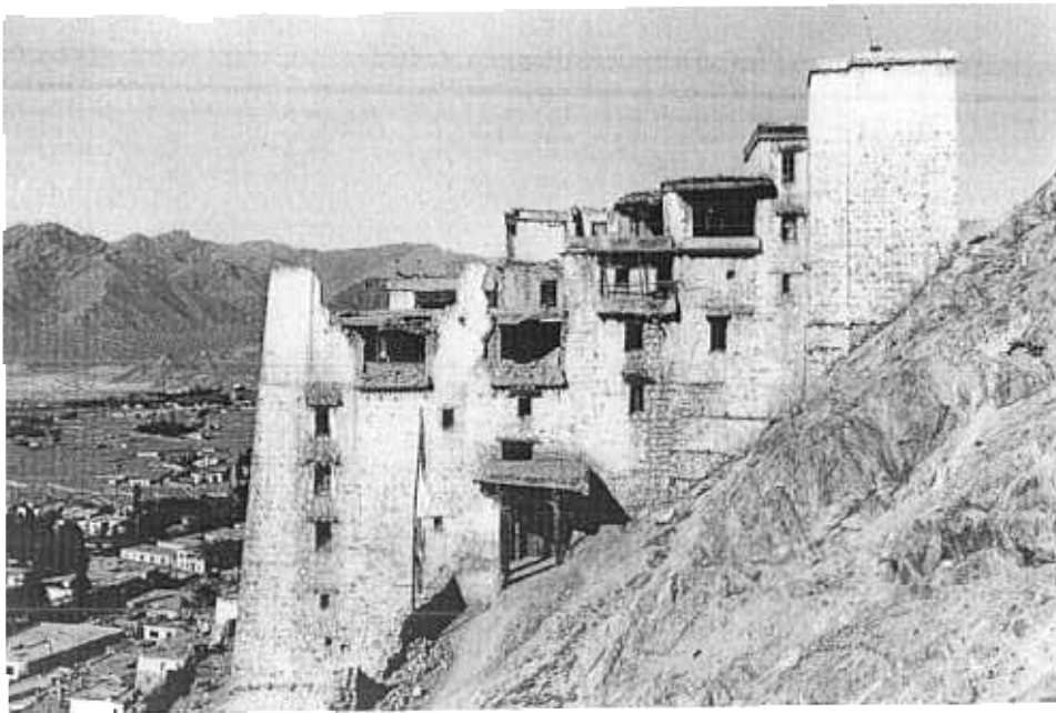
FIG. 16. The east elevation of the palace, showing the present condition. Note the majority of the collapsed sections are built of sunbaked bricks. ( Photo by John Sanday. )
