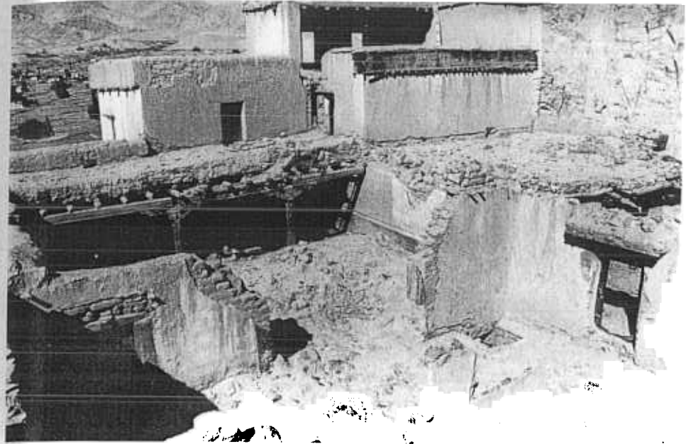
FIG. 17. The north-east corner from level 7 looking into Sangyeling temple, now collapsed. The construction at this level is in sunbaked brick, and its dilapidated state is due to neglect and severe weather conditions. ( Photo by John Sanday. )
