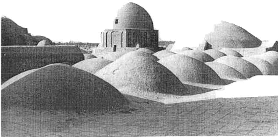
FIG. 8. Isfahan, Iran. The sequence of brick vaultings and domes in the Friday Mosque, before restoration.
