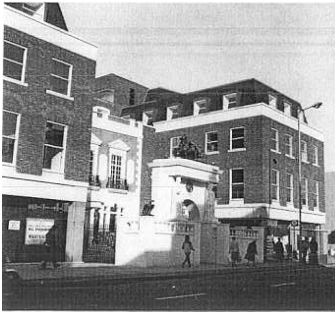
FIG. 7. The Pheasantry, King's Road, Chelsea, London, UK. The old facade propped up, the new bland and mediocre so as not to offend. This is, unfortunately, the growing trend in conservation.
