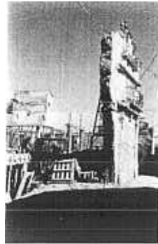
FIG. 6b. Conservation in Ejica, Spain. A fragment of facade propped up for incorporation into a new building. Is this conservation?
