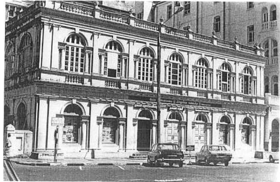
FIG. 2. Ministry of Information, Prince Street.
