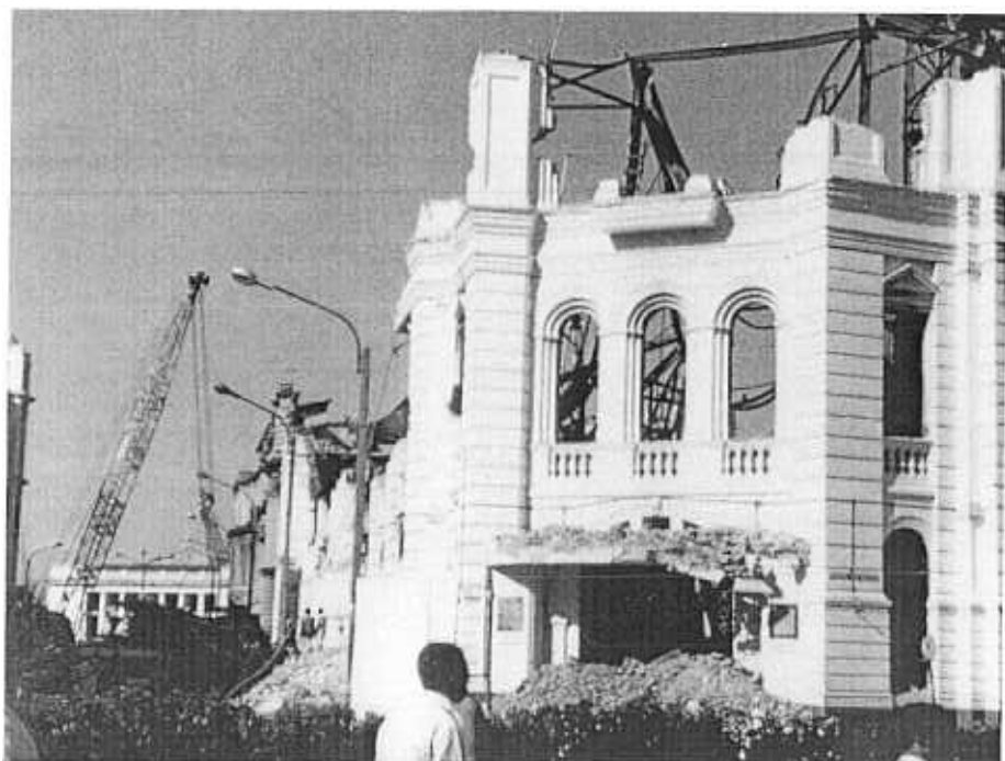
FIG. 1. The demolition of the fire-damaged Grindlays Bank, York Street.
