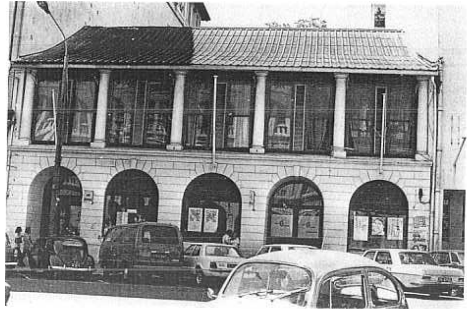
FIG. 4. Air Lanka office, Prince Street. A late eighteenth or early nineteenth-century building in which the arcade and colonnade were probably open originally.
