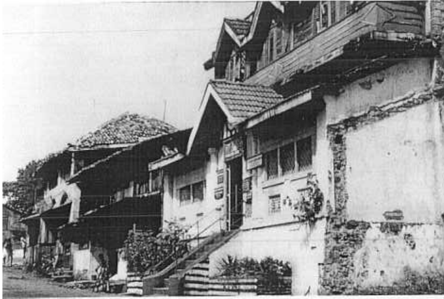
FIG. 13. Buildings at the corner of Mihindu Mawatha and St. Sebastian Hill.
