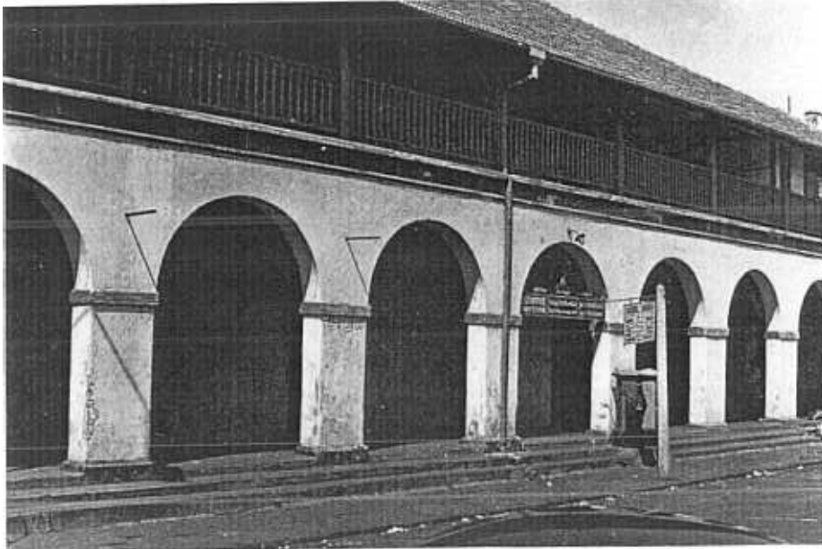
FIG. 5. The Post Office, First Cross Street. This was a draper's, F. X. Pereira's, from 1905 until about ten years ago. The building probably dates from the late nineteenth century.
