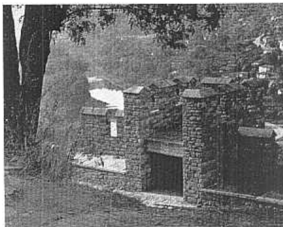
10. Tsarevets a view to the fortress wall after restoration
