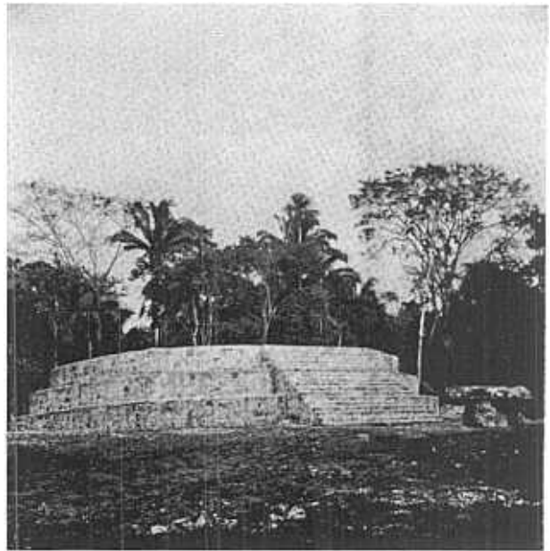
Fig. 14. — Looking southeast at Structure 79 after reconstruction. Notice jaguar altar in front of stairway.
