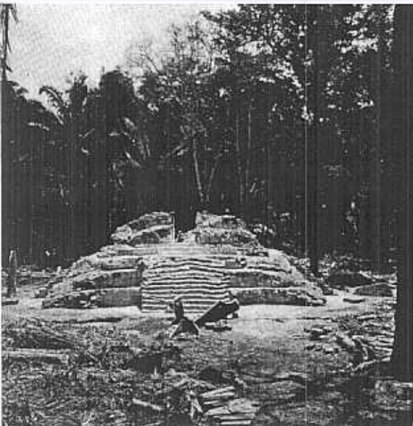
Fig. 3. — West side of Structure A-3 at end of excavation.
