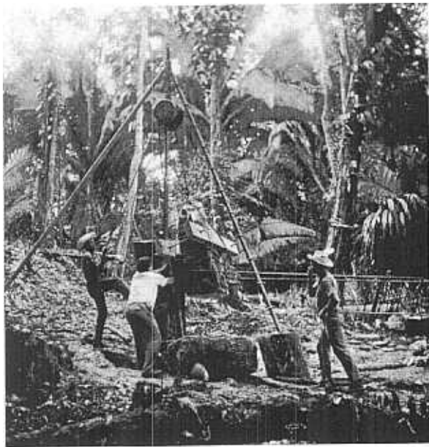
Fig. 18. — Erecting and mending Stela 2.
