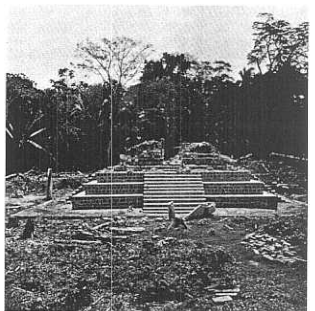
Fig. 4. — West side of Structure A-3 during reconstruction.
