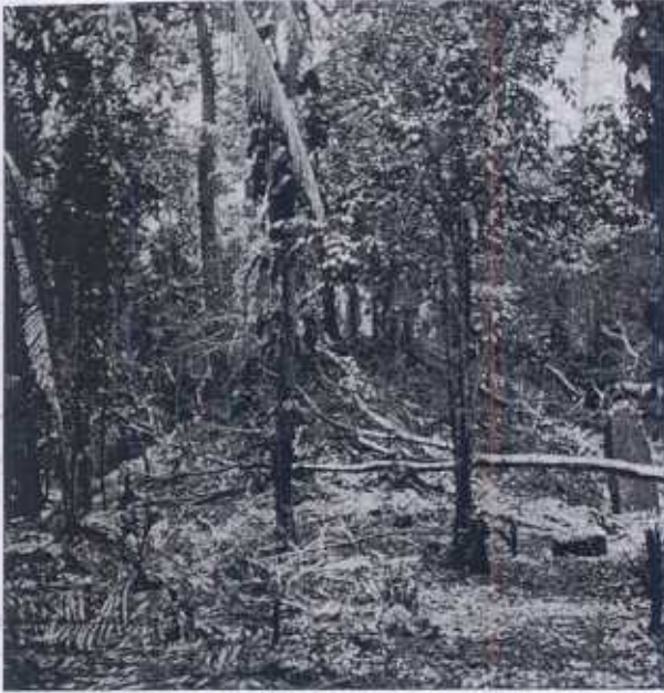
Fig. 1. — Northeast corner of Structure A-3 before excavation.
