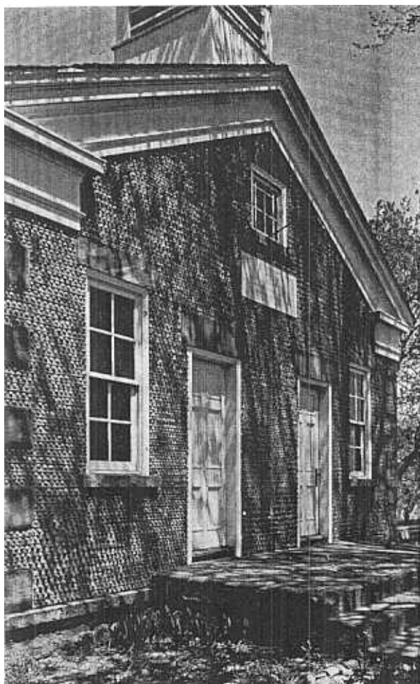
Fig. 12. — Cobblestone Schoolhouse (1849), District No. 5, Childs, N.Y. Architect: William J. Babbitt. Owned by Cobblestone Society of Childs, N.Y., open to the public as a District School House Museum. (Credit: National Park Service - Historic American Buildings Survey.)
