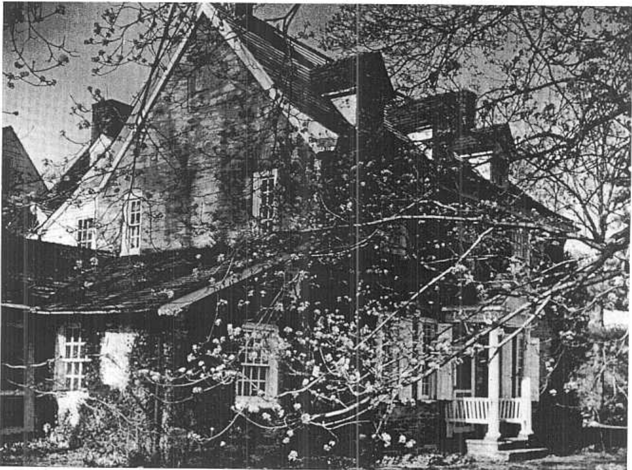
Fig. 9. — Harriton House (1697), Montgomery County, Pa. Built as the home of Charles Thomson, a signer of the Declaration of Independence. A $ 114,750 grant under HUD's Open Space Land Program was granted to purchase 14.6 acres of land, including the Harriton House which will be restored.
