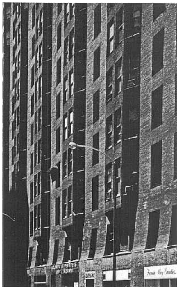
Fig. 15. — Monadnock Office Building (1891), Chicago, Ill. Architects: Burnham and Root. Designated by the Commission on Chicago Architectural Landmarks: « In recognition of its original design and its historical interest as the highest wall-bearing structure in Chicago. Restrained use of brick, soaring massive walls, omission of ornamental forms, unite in a building simple yet majestic. » (Credit: National Park Service - Historic American Buildings Survey.)
