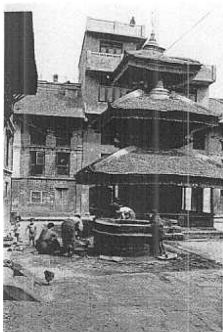
3. - Small public square in the NE sector of the Monument Zone. The disruptive tall building is of recent date.
