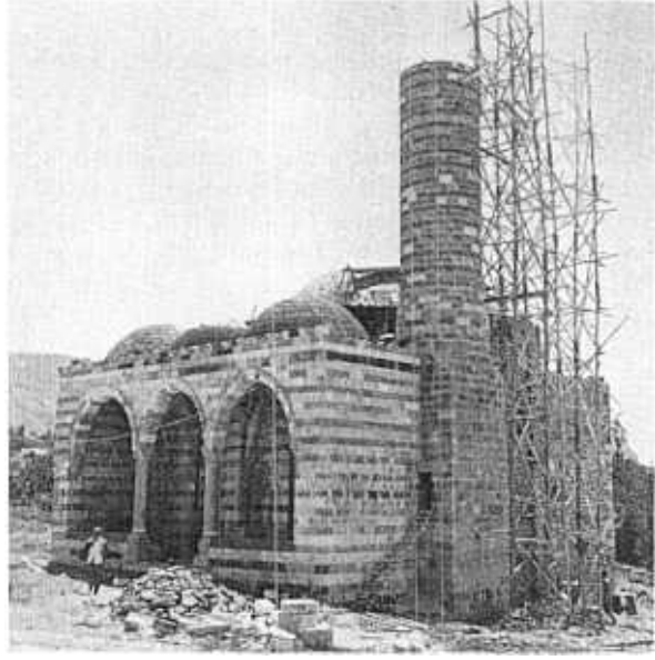
Fig. 7. - Reconstruction of the Baysungur Mosque at its new location in Yeni Pertek - southeast view.
