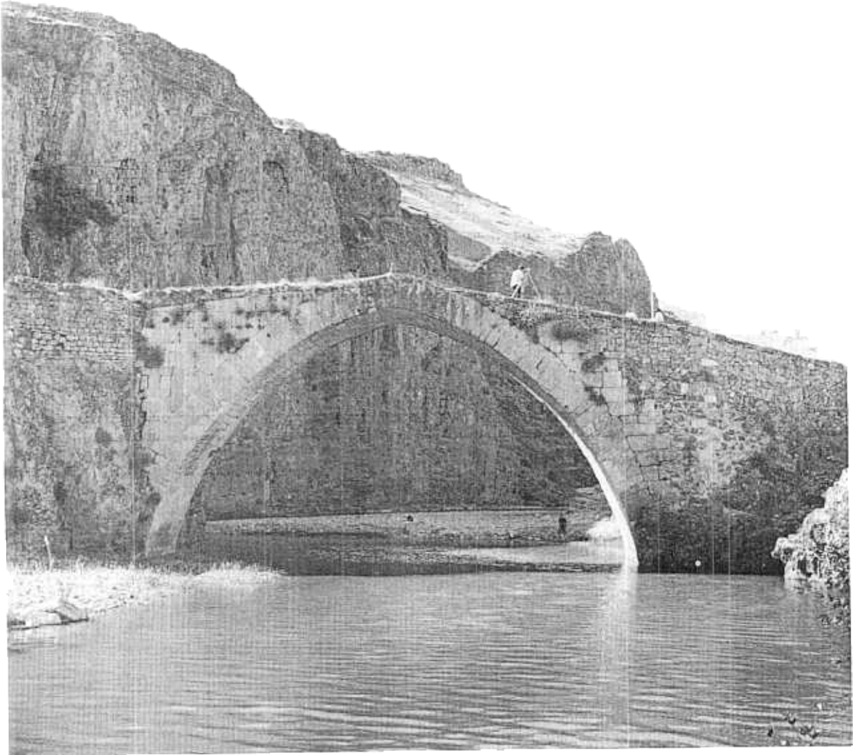
Fig. 10. - Recording the Karamağra Bridge prior to transport.
