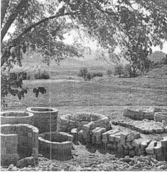
Fig. 6. - The minaret of the Çelebi Ali mosque (1567-1573) in Eski Pertek as dismantled for relocation.
