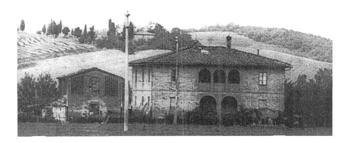
mixed brick and stone walls are frequent. Laterite is widely used for arches and vaults, and roofs are generally tiled.
