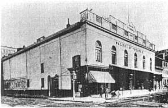
Fig. 7. - Walnut Street Theatre. Late nineteenth-century rusticated marble veneer and the niches at each end of the building have been replaced by storefronts. Courtesy of the Free Library of Philadelphia.
