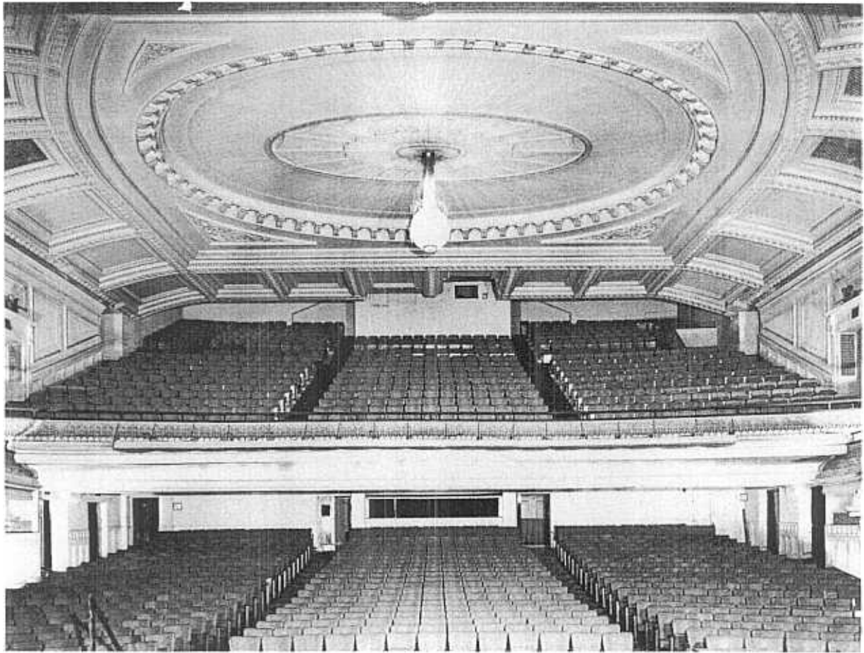
Fig. 16 The new cantilevered balcony built in 1920 replaced the 1828 balconies supported by cast iron columns (photo: Jack Boucher).
