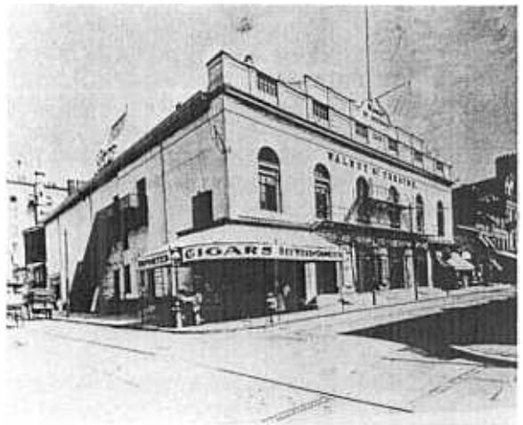
Fig. 9. - Walnut Street Theatre, ca. 1903. Fire-escapes have been added to both façades of the theatre. Courtesy of the Free Library of Philadelphia.
