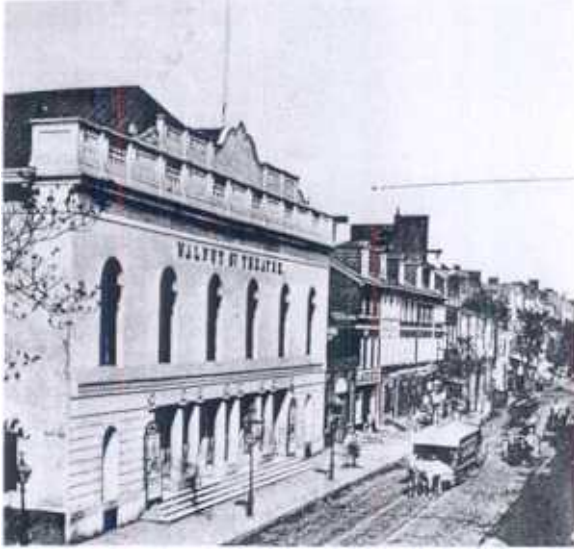
Fig. 6. - Walnut Street Theatre after the 1865 renovation. The Ninth Street wall has been raised, the cornice on Walnut Street has been replaced, the standing lamps have been removed and the porch floor has been lowered. Courtesy of The Library Company of Philadelphia.
