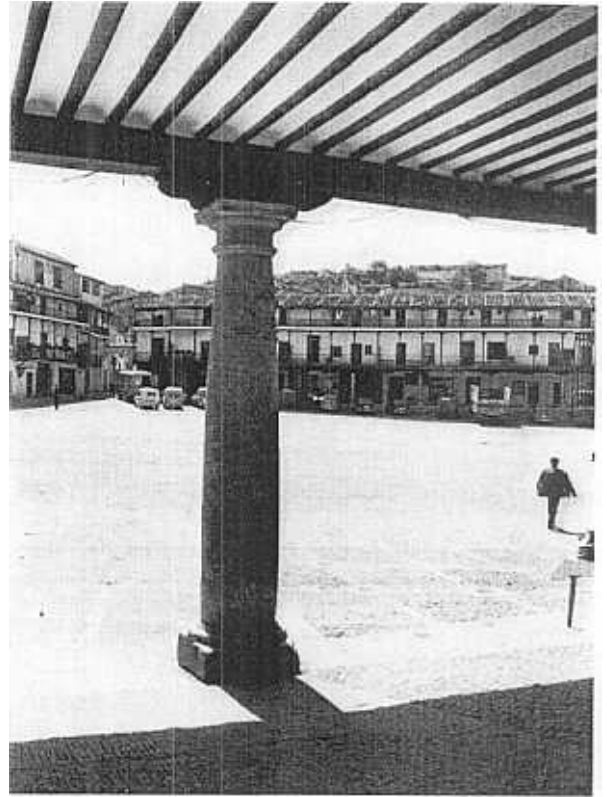
Fig. 5. — The Plaza seen from the bottom of the way up to the church, with detail of colonnade.
