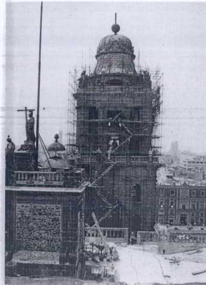
FIG. 1. Restoration being carried out on the West Tower.
