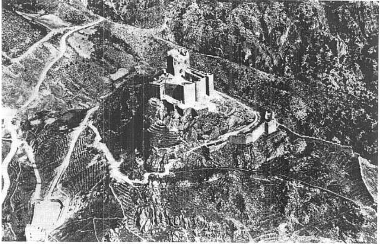
Fig. 3. — The castle enclosure during restoration, aerial view.
