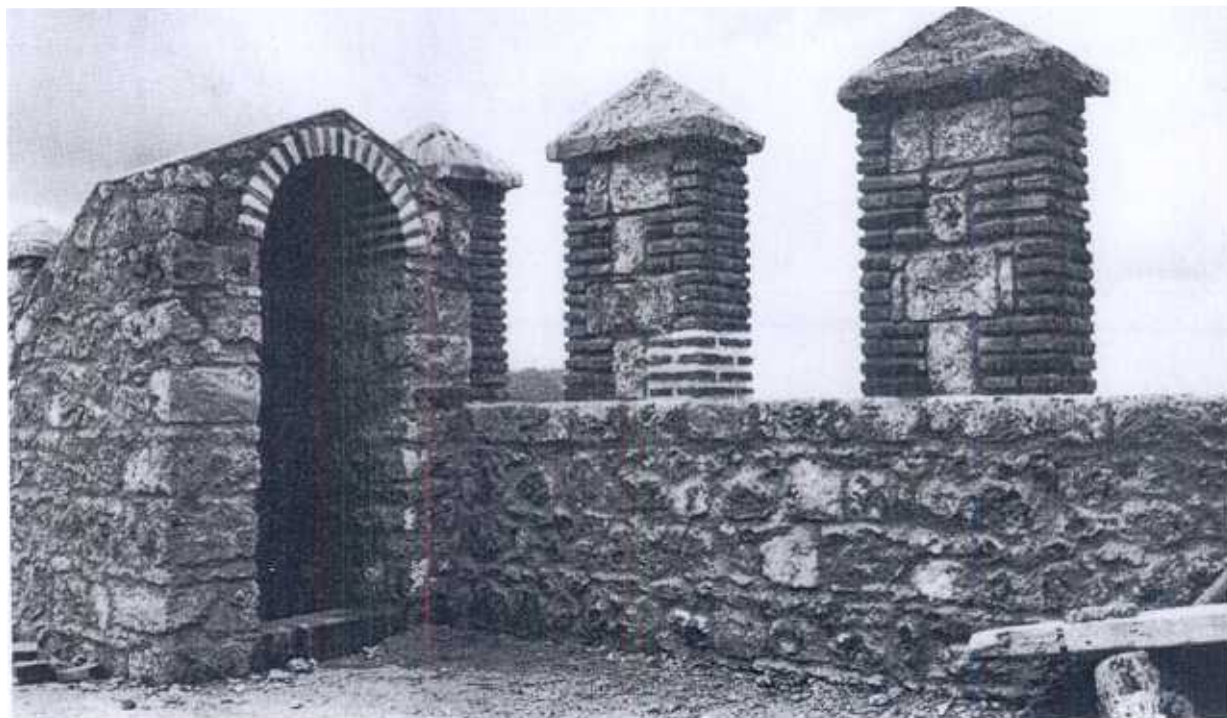
Fig. 8. Crenellations and staircase entry (detail), at top of tower.
