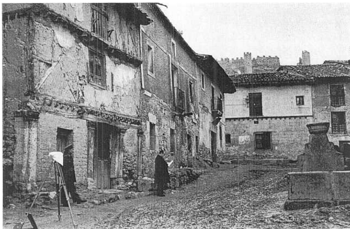
Fig. 1. — The Town Hall Square, condition when work started.
