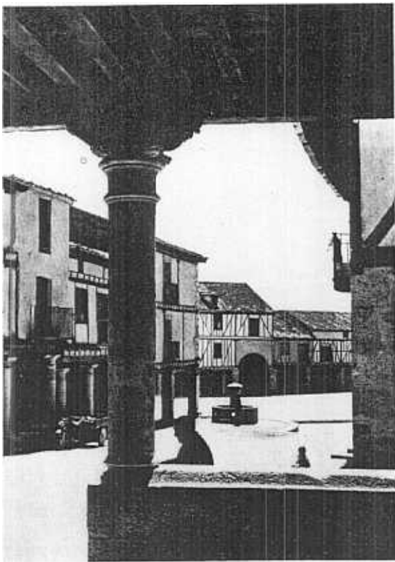
Fig. 2. — The monuments as they appeared during the renovation work. In the background, the Castle and the Town Hall with the porch of the latter partially uncovered.
