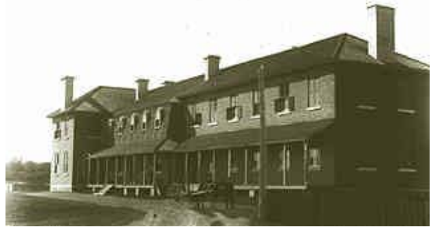
Figure 6 The New First Class Hotel. Parks Canada.
