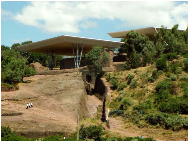
Figure 1 Temporary shelters to protect the churches from rainfall and erosion. E. Negussie, 2009.
