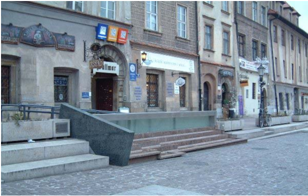
Figure 4 A highly inappropriate modernist fountain on Mały Rynek located within the World Heritage site. M. Taylor, 2009.
