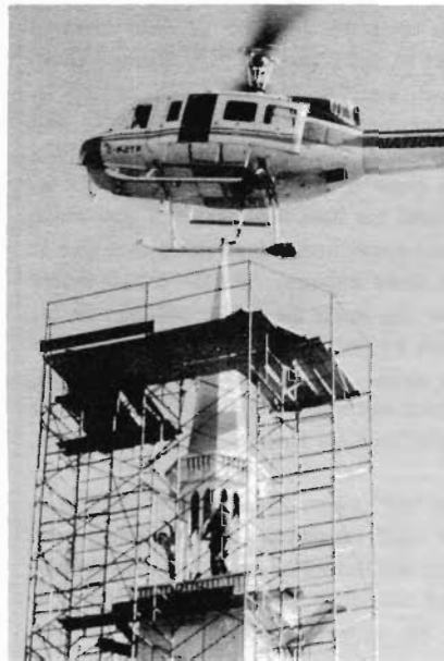
The replica spire was airlifted into place.
