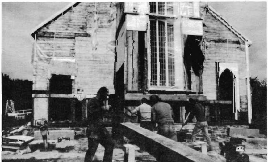
Indian people from the Stanley Mission reserve restoring heavy timber frames.
