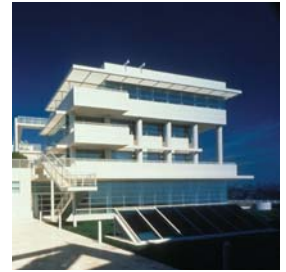
Getty Center East Building is GCI's headquarters
