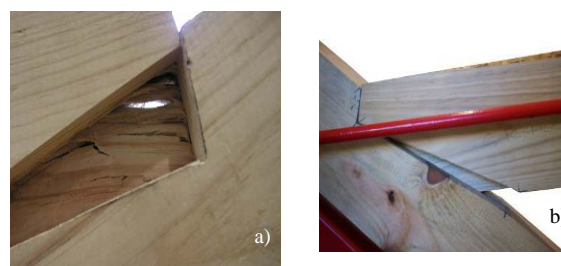
Figure 17. a) Failure in the tenon (closing skew angle); b) deformed shape (opening the skew angle)
