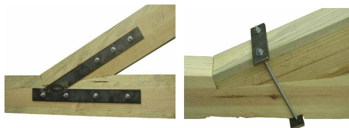
Figure 6. Stirrups and tension ties
