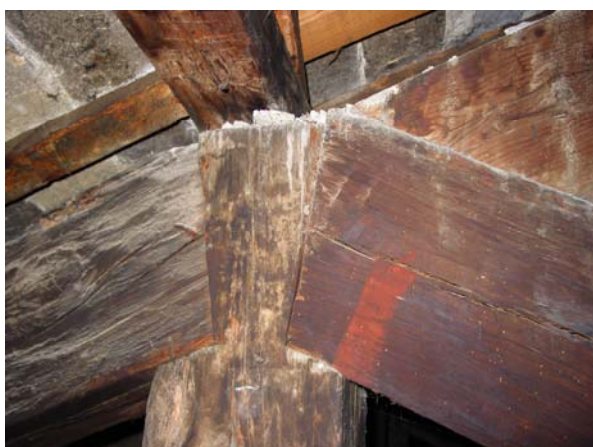
Figure 3. Joints details. Conjunction between the knee rafters and the king post. (N. Lombardini,
