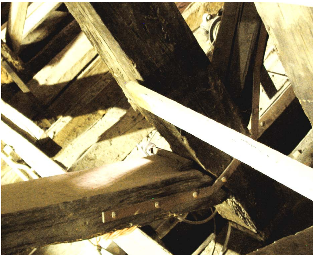
Figure 5. Examples of disjunctions between struts and king post at several trusses (N. Lombardini, 2007)
