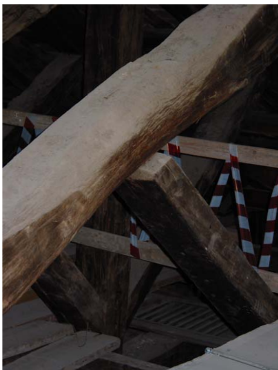
Figure 5. Examples of disjunctions between struts and king post at several trusses (N. Lombardini, 2007)
