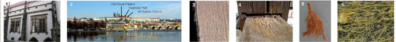
Figure 1 – View on the Vladislav Hall building. Figure 2 – View on Prague Castle. Figure 3 – fine fibers on wood surface has appeared again after conservation treatment. Figure 4 – The most damaged timber above the Vladislav Hall. Figure 5 – Detail of the corroded wood from the figure 4. Figure 6 – Fiber sample taken by tape from the wood surface.
