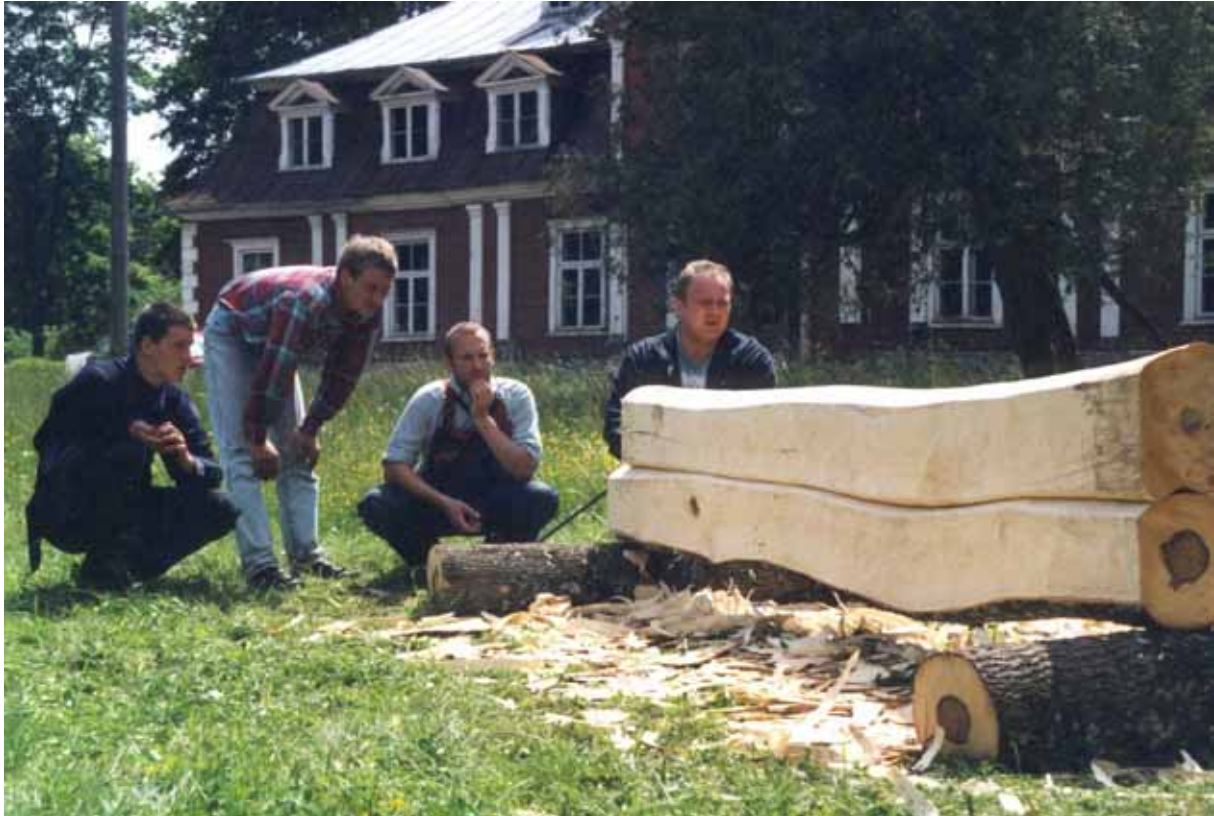
Fig 4. Workshop on the repair of timber; Ungurmuiza, Latvia
