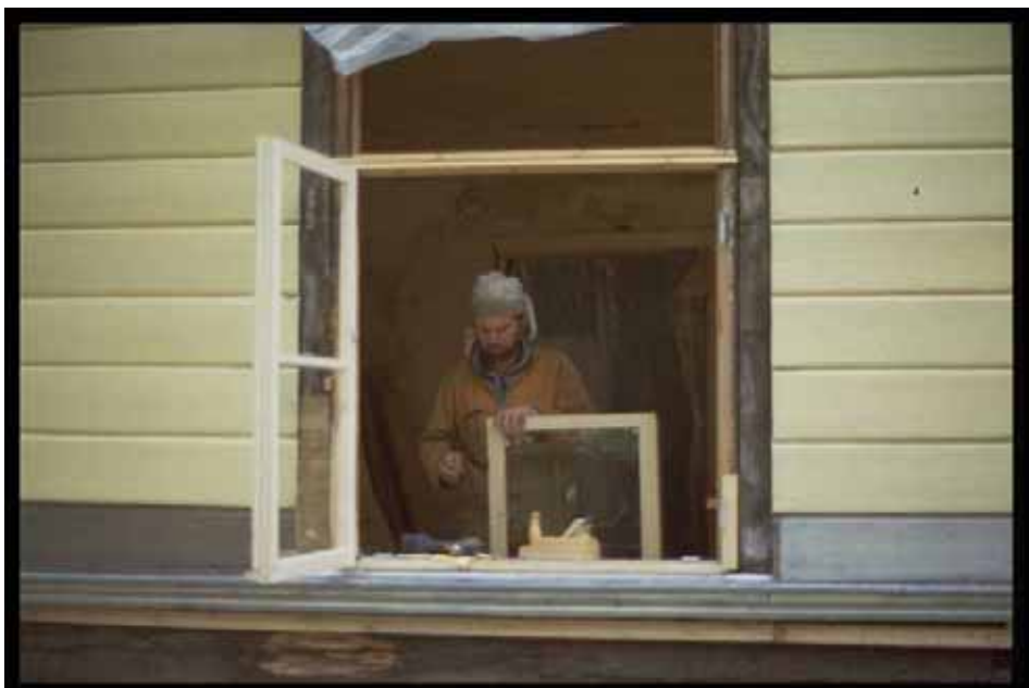
Fig 9. Workshop on the repair of windows, Tallinn, Estonia
