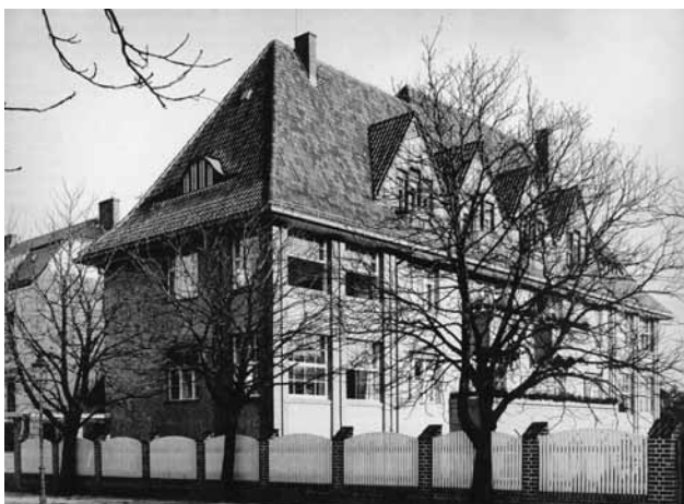
Fig. 1 Boardinghouse, Berlin-Westend, Kastanienallee 32, August Endell, 1908, street and garden facades
