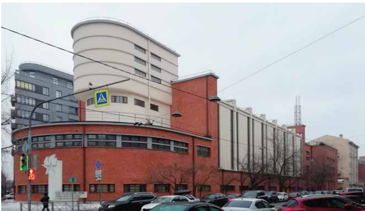
Fig. 7 Power station of the Red Banner factory, 2022
