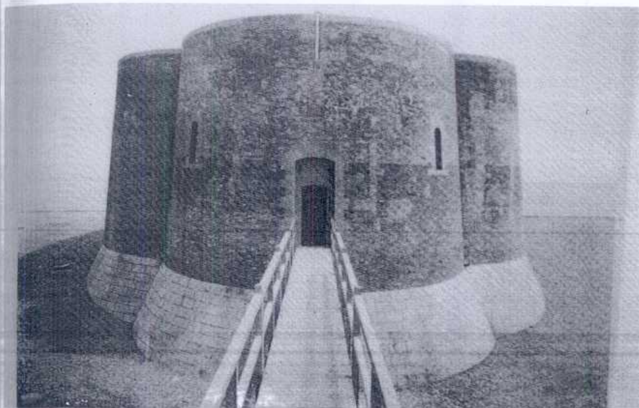
Curved and inward sloping walls in brick fortification. (Aldeburgh, England).
