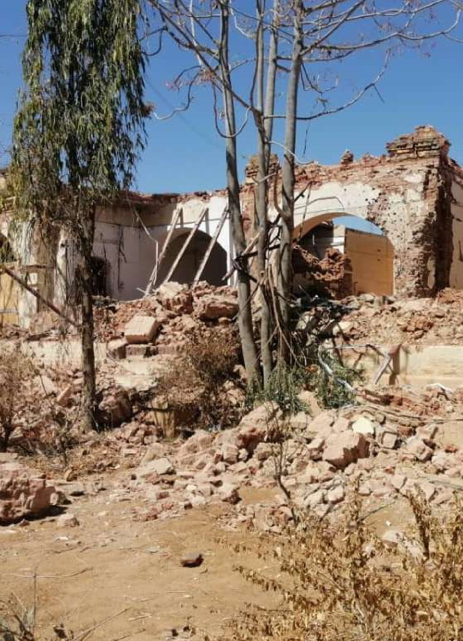
Collapse of the Directorate Building in El-Obeid city after it was hit by several shells
