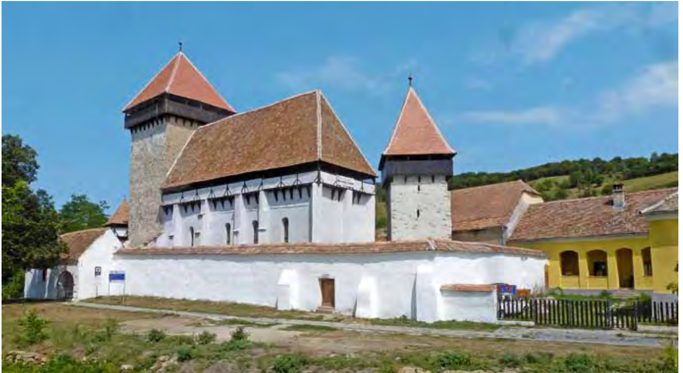
Stejăriș/Propstorf, fortress after the completion of the measure
