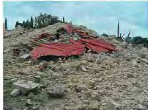
Loon and Maribojoc churches in state of rubble
