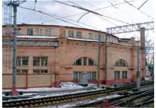
View of the Circular Depot today (© MAPS)
