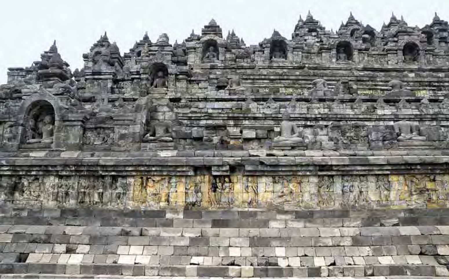
Temple front showing different types of decay
