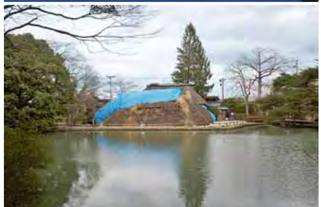
Yubikan, main building of the historic site, before the earthquake (top) and after (bottom)
