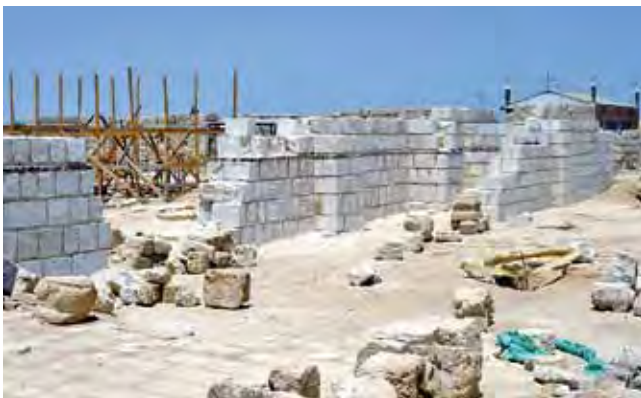
Abu Mina, recent "restoration" work using gypsum lime stones (photo: W. Mayer)
