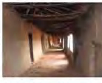
Photo 14. Internal corridor of the palace
