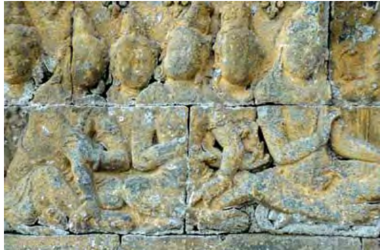
Detail of a relief showing severe rounding
