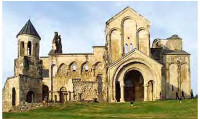
Bagrati Cathedral before the intervention (photo: www.monument.ge )
