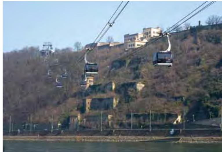
Cable cars connecting the city of Koblenz with Ehrenbreitstein fortress (photo: C. Machat)
