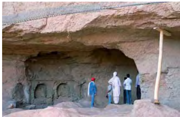
Parts of the niche's back wall had to be supported as stone slabs kept falling down
