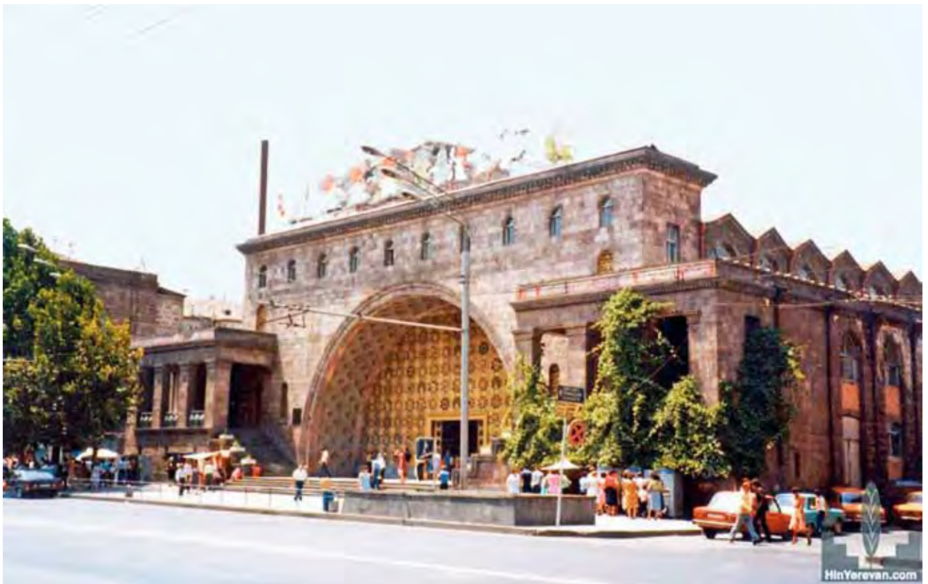
The Central Covered Market in 1985 (architect Grigor Aghababyan, engineer Hamazasp Arakelyan)
