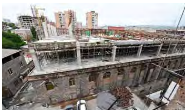
The new structures of the "renovated" Covered Market
