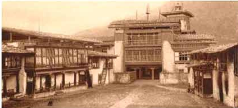
A photograph of the first courtyard (facing Dukhang building) taken in 1905
