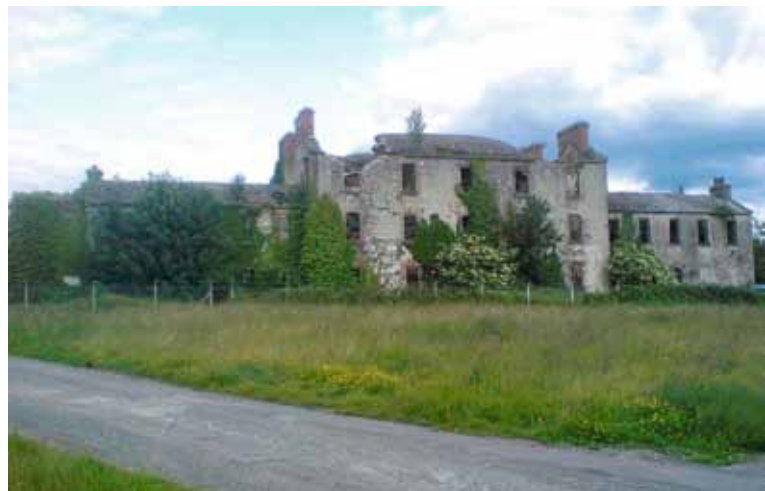
Former Military Barracks, Nenagh, Tipperary North, 2013
