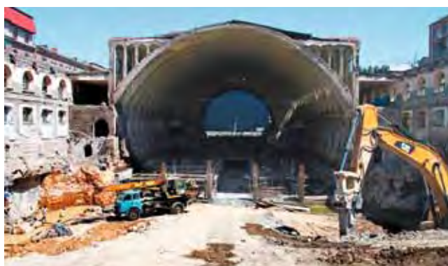
The demolition of the Covered Market started in 2012
