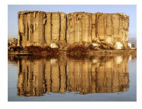
for over 20 days, with first minimal interventions to attempt to contain it apparently only taking place **after 10 days following widespread protest and calls for action by civil society.** This section of the silos had been tipping since the explosion in 2020, and could probably have been saved if timely action had been taken, but the fires further deteriorated the structure hastening its collapse.
